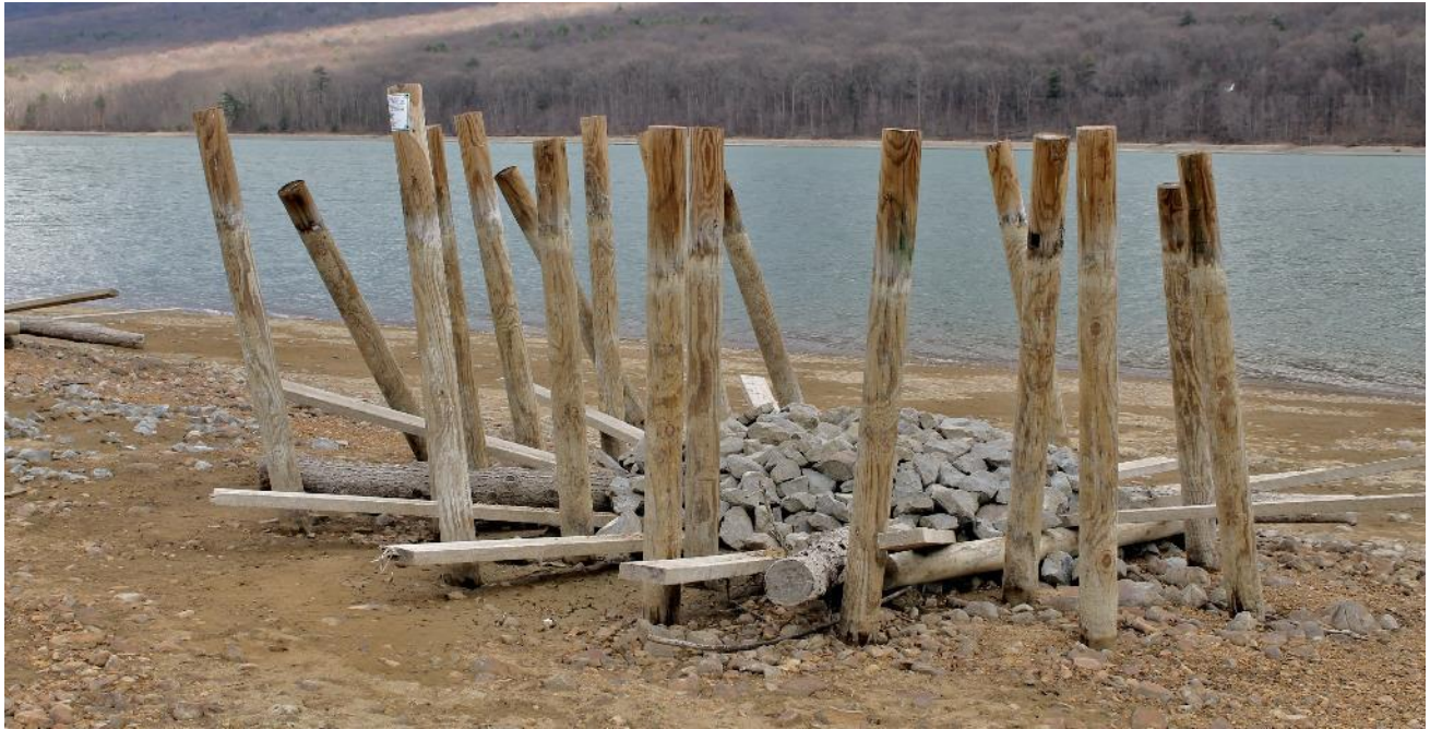
Figure 16 - Example Fish Habitat Enhancement Structure Ultimately Located on Bottom of Lake
